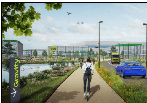
The Gravity site is under construction
